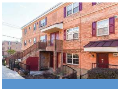
Villages at Parklands, Ward 8 Rehabilitation
