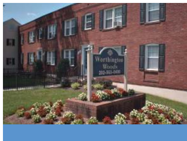
Worthington Woods Apartments, Ward 8 Rehabilitation
