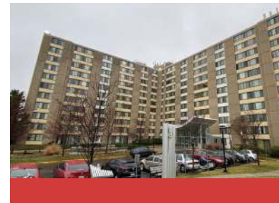
Edgewood 611/Edgewood Gardens Apartments, Ward 5 Rehabilitation
